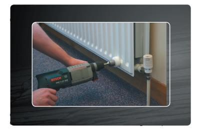
These deposits can, especially on older systems, become quite solid and stubborn to shift. To speed up the chemical flushing process and improve the cleansing efficiency it is recommended to vibrate the radiator surface to loosen the deposits within.
